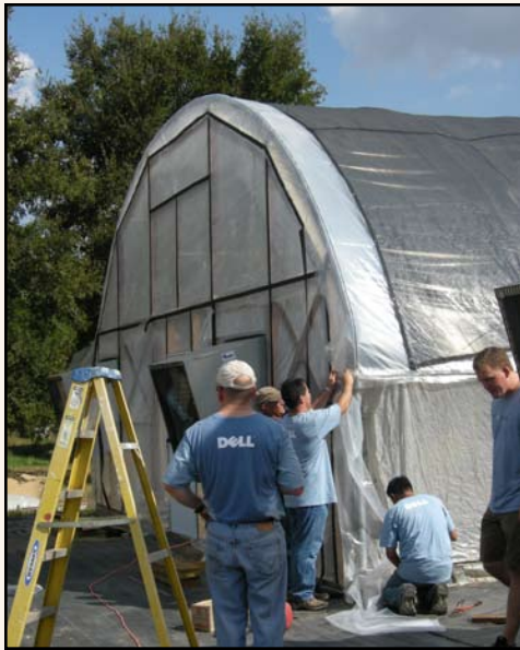
(Above) Dell volunteers putting new skin on the Llano greenhouses. Two layers of plastic are installed and then a pump blows air between the layers, inflating a space that helps keep the houses cooler in the summer and warmer in winter.
