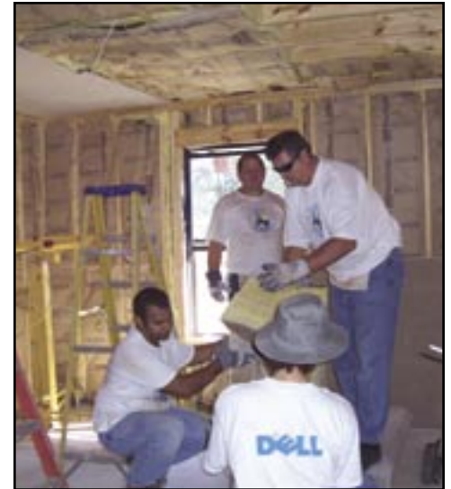
Dell employees work together on Jacob House, installing insulation and sheetrock.
