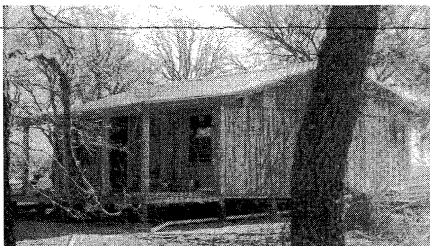
Cedar volunteer cabin under construction.
