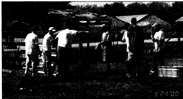
Students from St. Stephen's Episcopal School help clear rubble from the barn fire and set new temporary gates.
