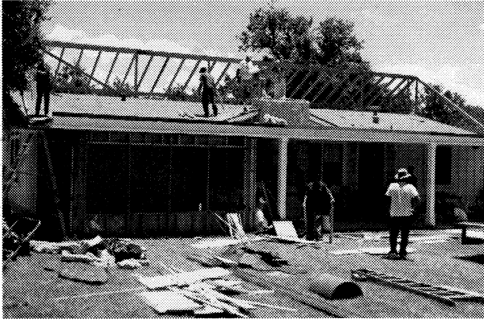
Roof trusses about to come down
