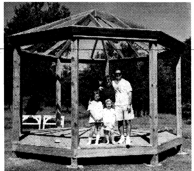
Dan, Sally, Jennifer & Janie Nowland inspect gazebo in early stages of being erected The gazebo is a gift to the Ranch in memory of baby Kelly Nowland
